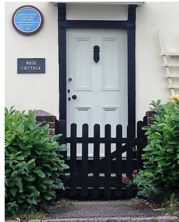
Photo 9. View of House Facade at Church End
